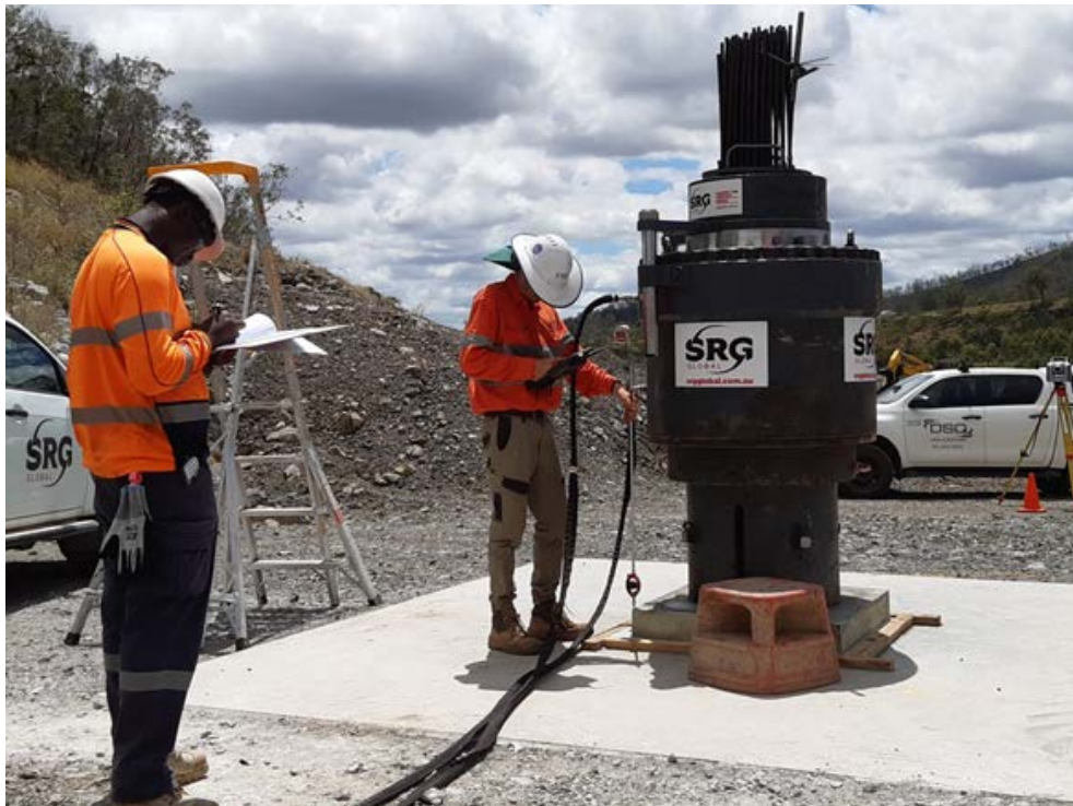
Figure 26 Anchors being stress-tested by 2,200t capacity jack at Paradise Dam (January 2021)
