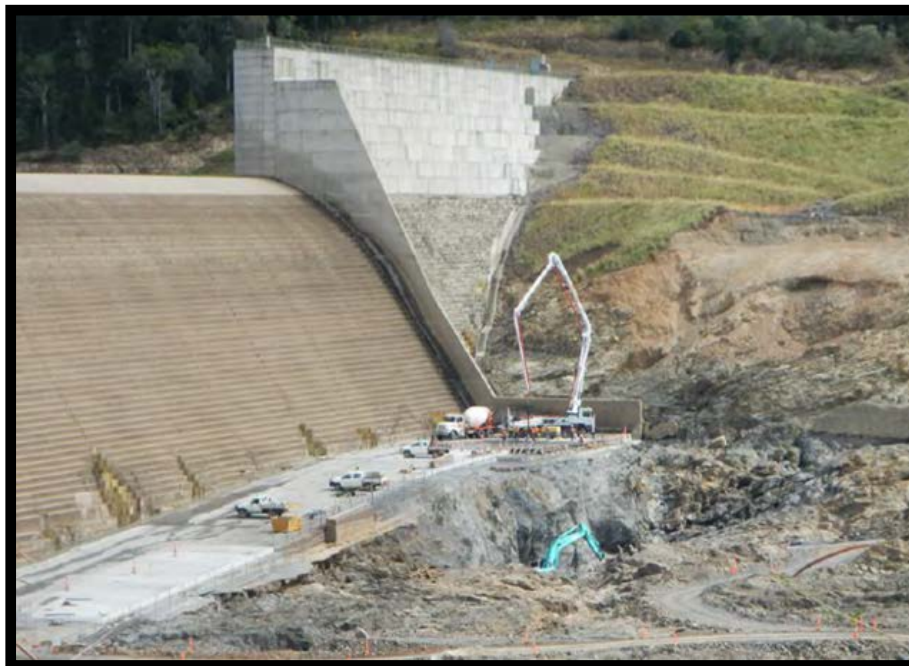
Figure 2 Scour damage at Paradise Dam
