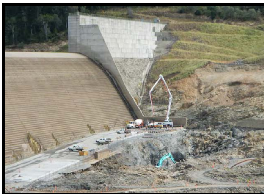
Figure 16 Scour damage at Paradise Dam
